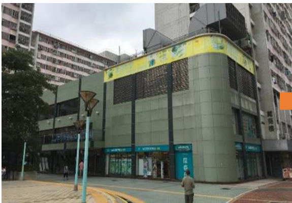
Lai Kok Shopping Center (Before)
